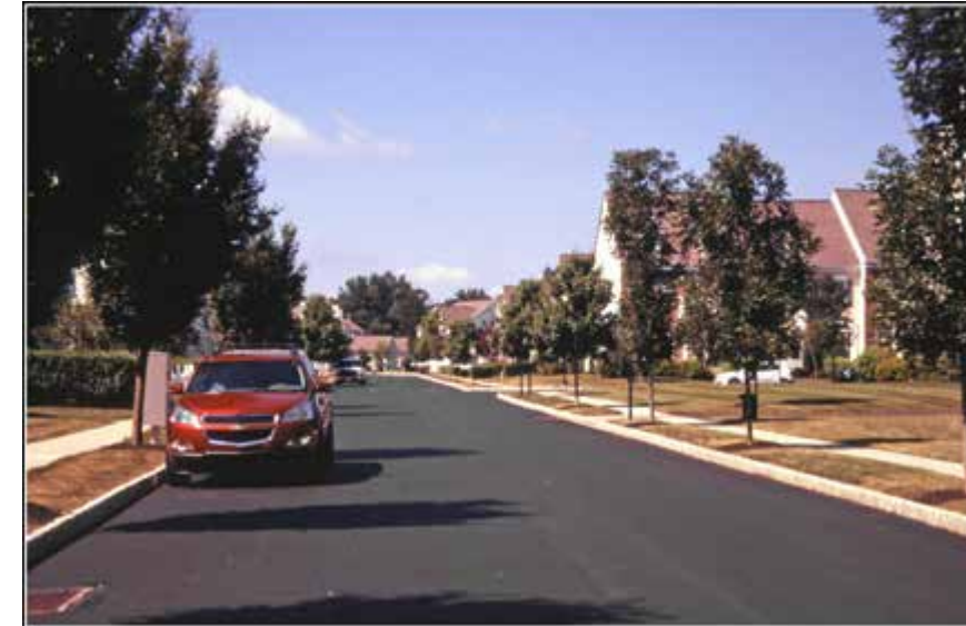
This road in Bedminster Square follows context sensitive principles. The road allows parking on one side. The width has been created so that two vehicles can simultaneously pass the parked vehicle but at moderate speeds. A wider road would allow passing at higher speeds, not a desirable objective in the TND.
