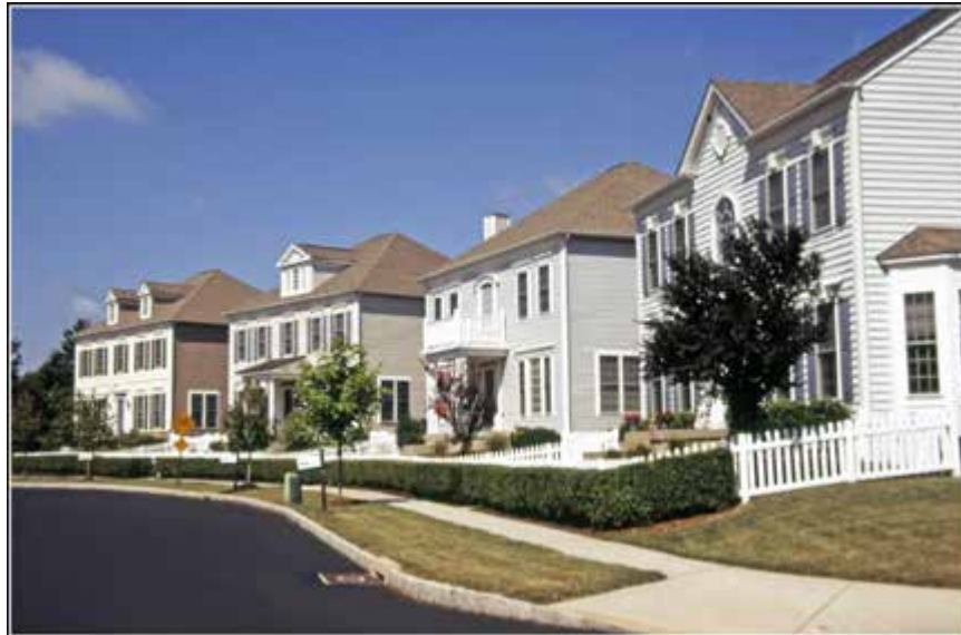
The dwellings in Bedminster Square are effectively arranged to create the street wall. Closer to the street, the fence and the hedges create a secondary street wall.
