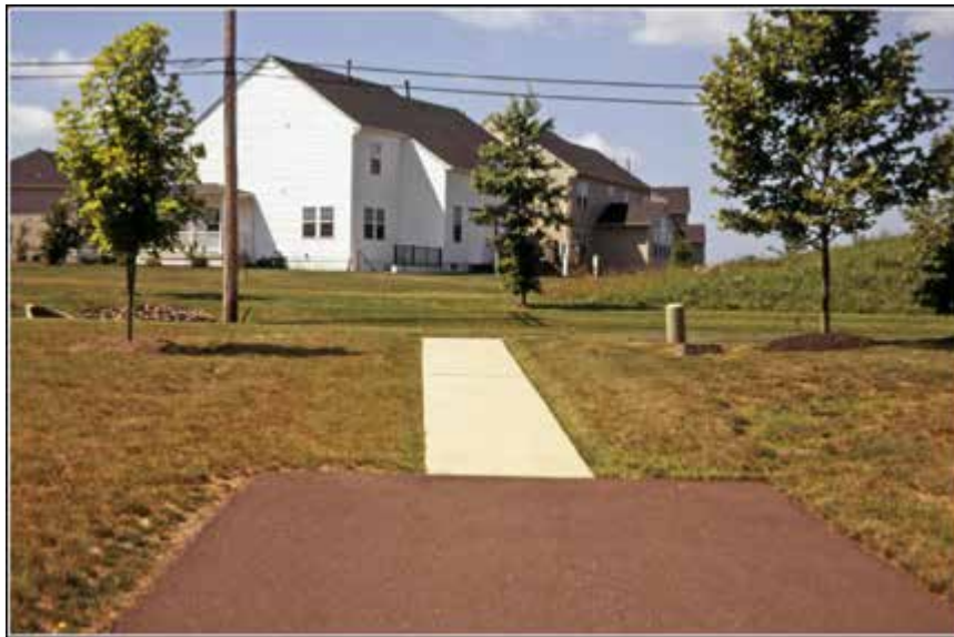
Bedminster Hunt West provides this pedestrian shortcut at the end of an alley.
