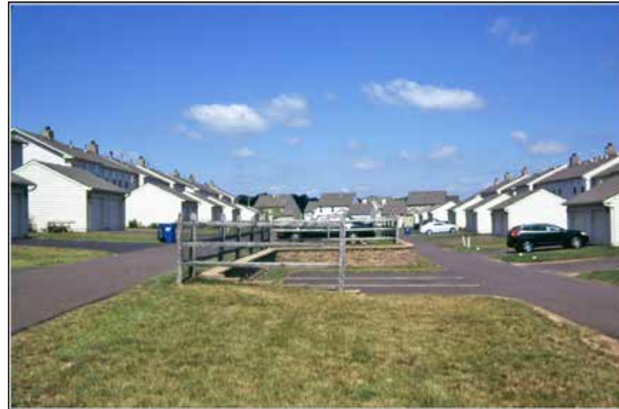
Bedminster Hunt West features an elaborate alley between two rows of townhouses. The alley occupies an area forty feet in width. Two travel lanes are provided. Interestingly, both travel lanes offer one-way travel in the same direction. A parking area is found in between the two travel lanes. The parking area is provided in addition to private garages.
