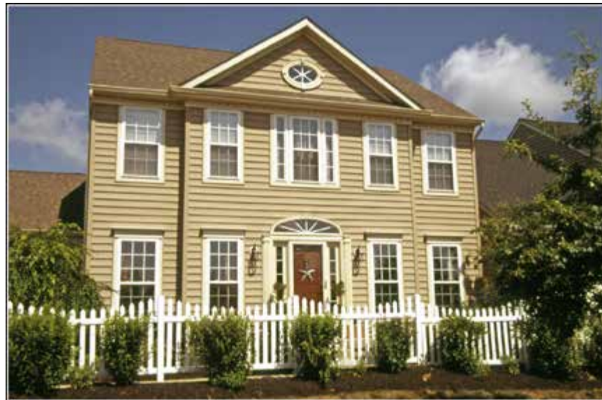
TNDs feature architectural styles not typically found in current construction. The windows are prominent in this example from Bedminster Hunt West.
