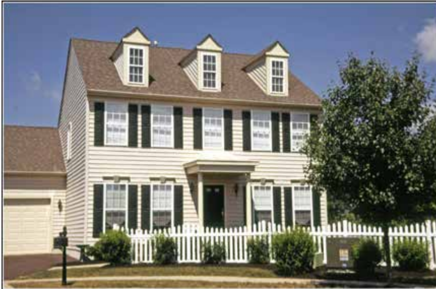
The architecture found in TNDs like Bedminster Hunt West is derived from features found in historic styles.
