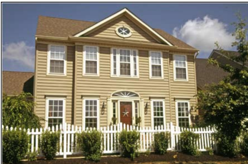
TNDs feature architectural styles not typically found in current construction. The windows are prominent in this example from Bedminster Hunt West.
