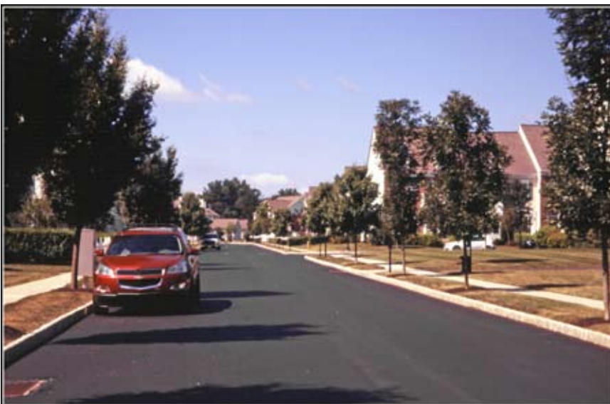
This road in Bedminster Square follows context sensitive principles. The road allows parking on one side. The width has been created so that two vehicles can simultaneously pass the parked vehicle but at moderate speeds. A wider road would allow passing at higher speeds, not a desirable objective in the TND.
