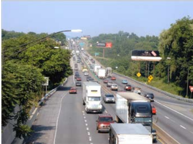
Route 22 looking east toward Lehigh River Bridge
